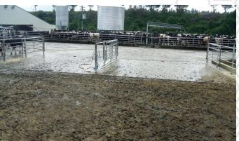
Entry to the milking shed showing a smooth & pothole free transition from race to concrete after 8 months usage.
